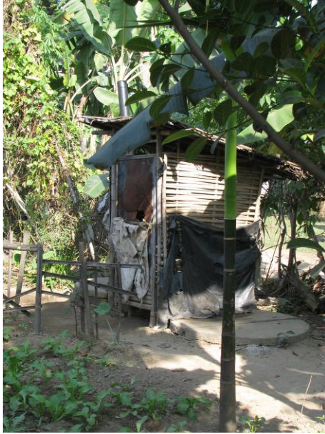
Toilet facilities are shared by two huts.
